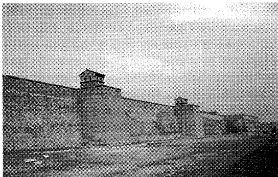
Fig. 9 'Horse faces' on wall of district headquarters, Pingyao, Shanxi
