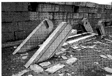
Fig. 14 ‘Suspended gate’ of Pan Gate, Suzhou, Jiangsu
