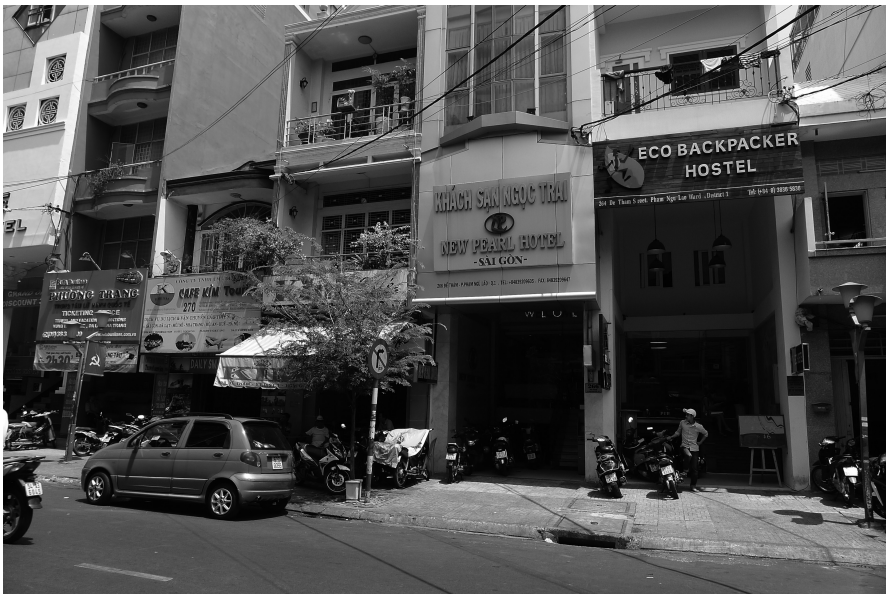
Fig. 6. Street scene along Đề Thám Street (east side)
